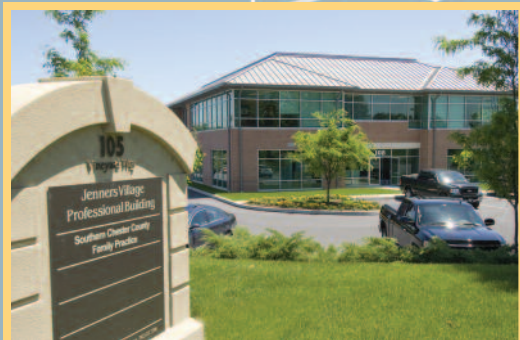
WEST GROVE MEDICAL BUILDING
